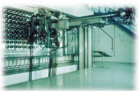
Fuelling machine in operating position at face of reactor.
